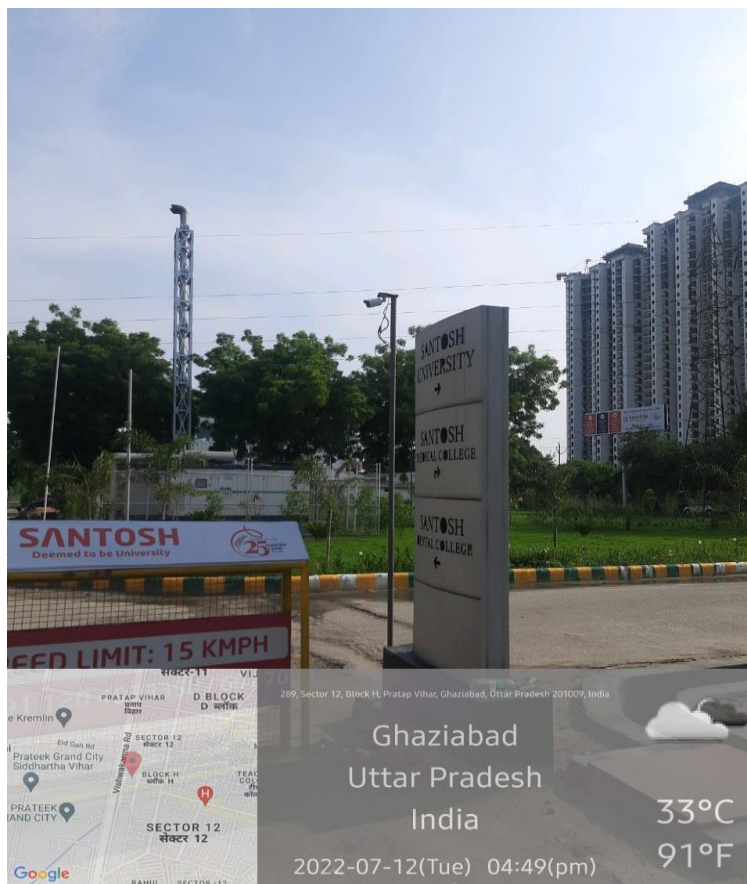
Campus CCTV Camera Surveillance
